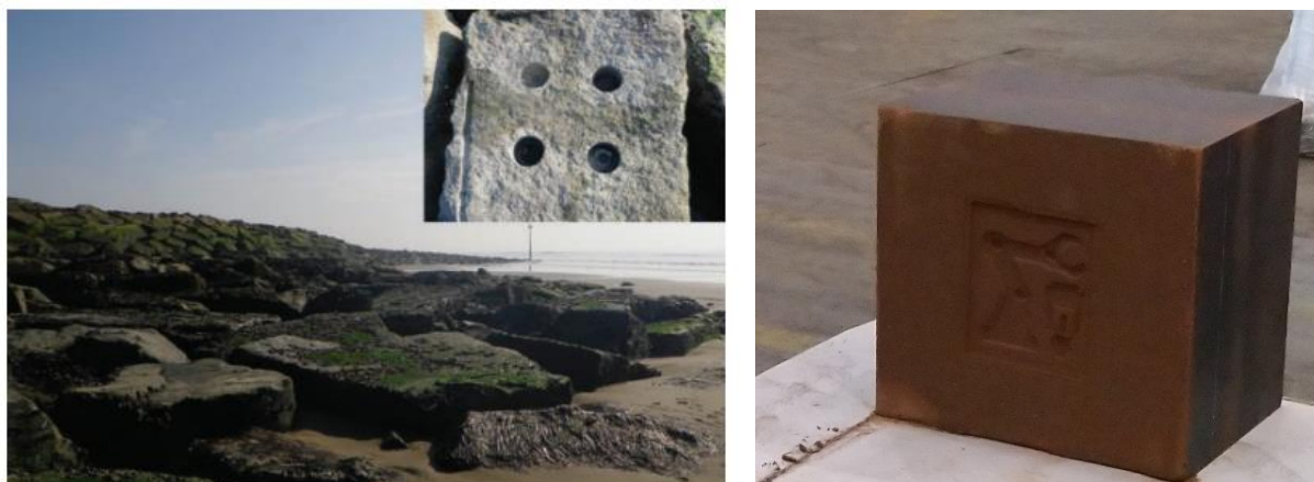
Figuur 3-9 Links: Theekop holtes in oeververdediging (Evans et al., 2016). Rechts: structuren in GEOWALL®-persproces
